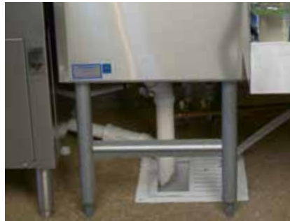
Place, level & plumb.
